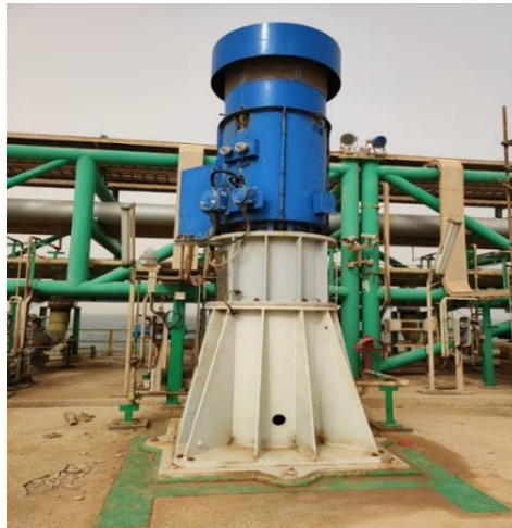
Fig. 18. Sea Water Intake Pump
