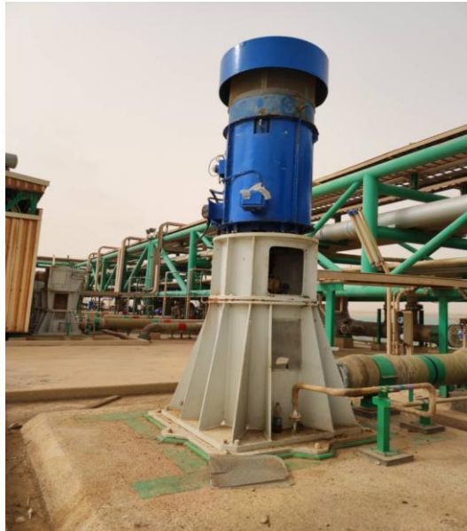
Fig. 9. Sea Water Intake Pump
